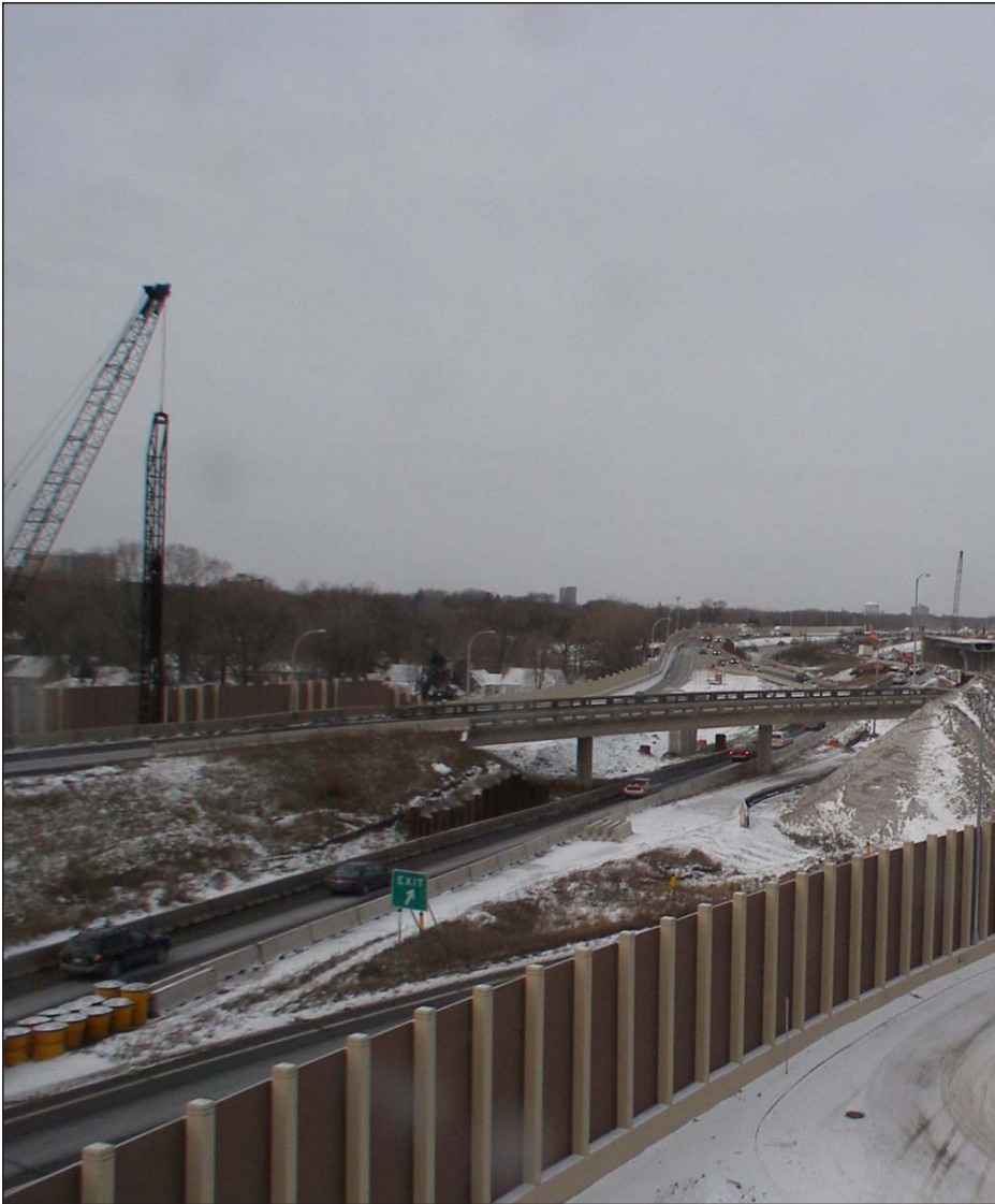
Pile driving continues on the 35W/Crosstown
